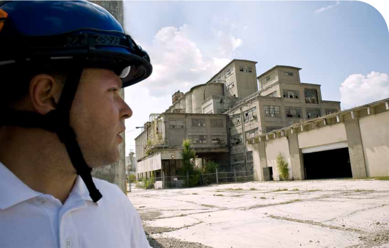
Mark Gebhart surveys the former CEMEX concrete plant, a 54-acre property that will be transformed into the National Center for Medical Readiness (NCMR). Gebhart serves as NCMR’s director.
